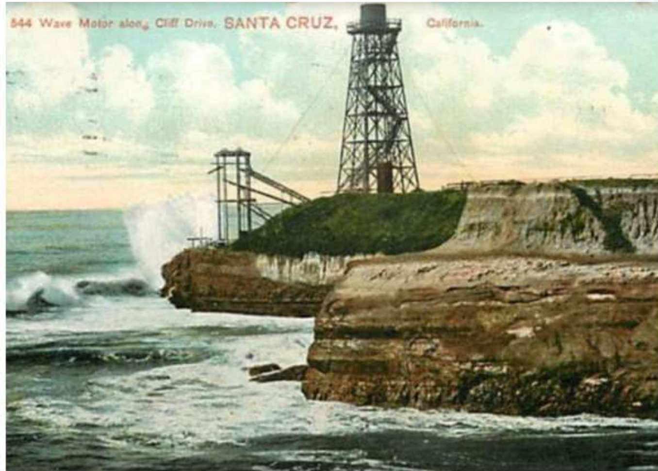
Postcard from a “wave motor” experiment off the coast of Santa Cruz from 1898 (Budal and Falnes, 1975)
